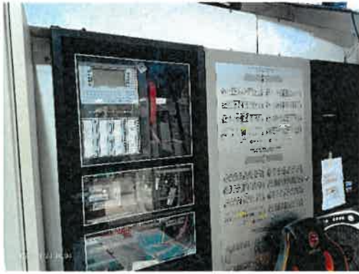
fire alarm control panel
